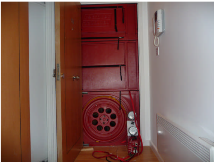
16. Applying negative air pressure
