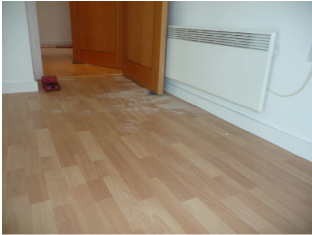
22. Showing dust entrainment under negative pressure
