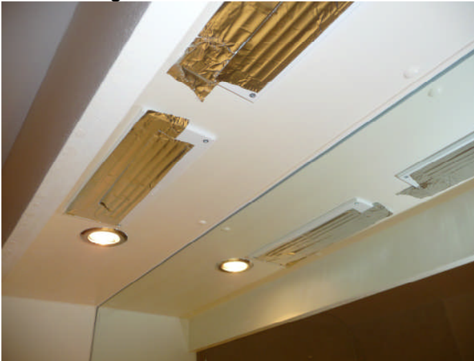
15. Sealing vents and holes prior to application of negative air
