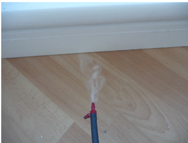
24. Showing chemical smoke being sucked out under windows under positive pressure
