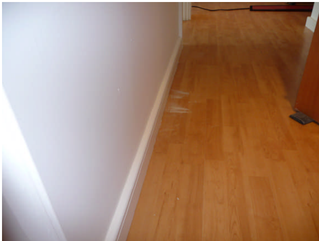
23. Showing dust entrainment under negative pressure
