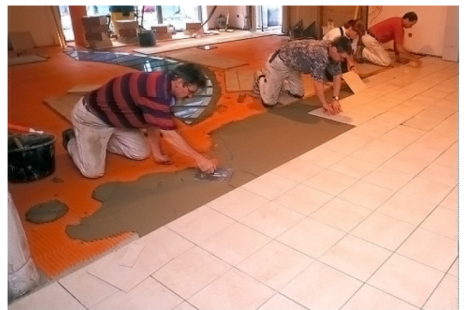
Photograph 11: Tile Installation
