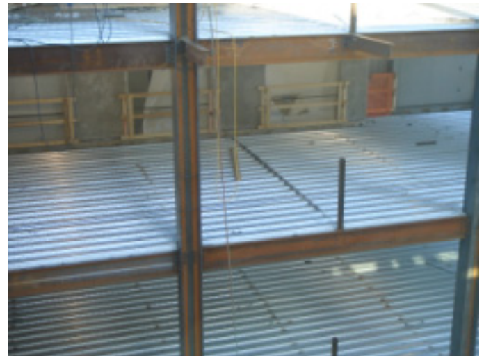
Photograph 6: Fluted Steel Deck
