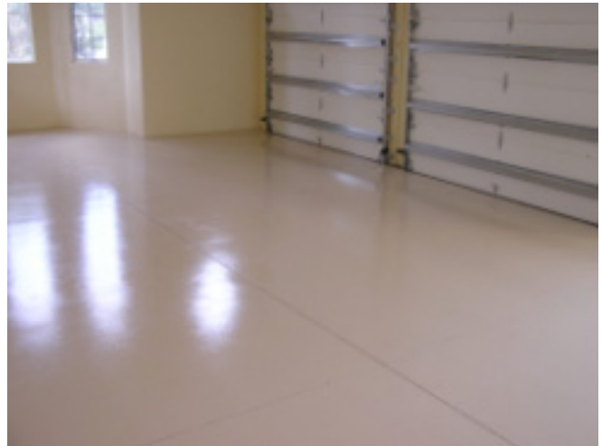
Photograph 7: Epoxy Coatings
